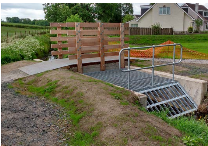
New footbridge and trash screen, with bunded storage area in background.
