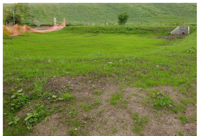
New bunded storage area and outlet back into watercourse.
