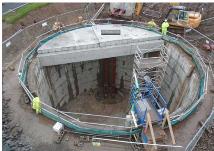
Storage tank at Moraine Avenue under construction
