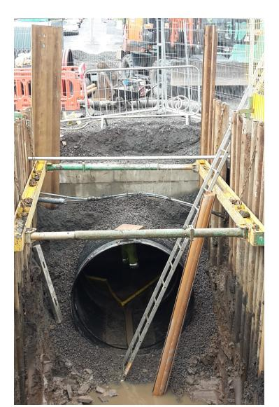
Manholes are constructed along at each change in direction of the pipework.
